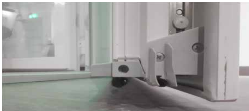
Retractable floor sealing mechanism at the bottom part.
